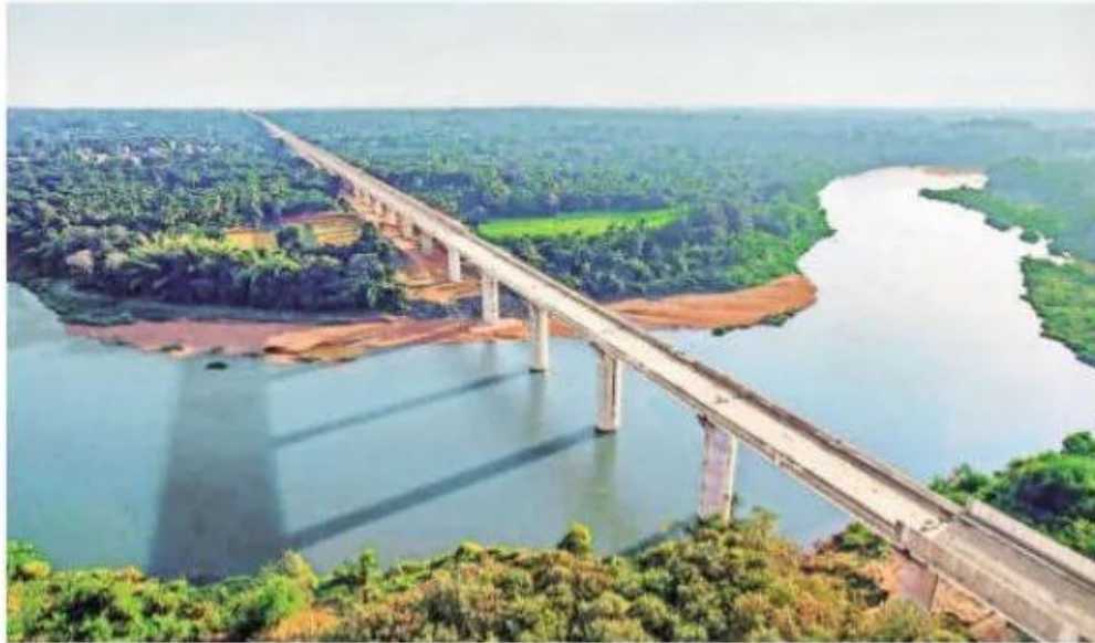
An aerial view of India's first Bullet Train corridor between Mumbai and Ahmedabad after completion of 300 km of viaducts, on Tuesday. ANI
